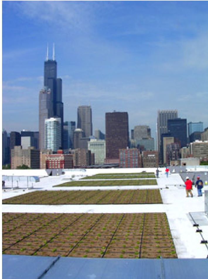
Figure 12: Extensive Green Roof System [5].
